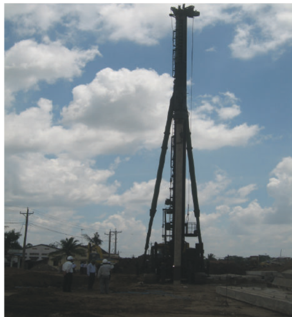
打桩机 Pile driver
