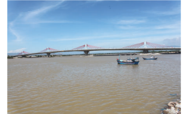
Investor: Department of Transport of Ninh Thuan Province Project name: Coastal Road of Ninh Thuan Province Contract price: 386,981 million VND Year of implementation: 2012 -:2015 Road bridge project, level I
