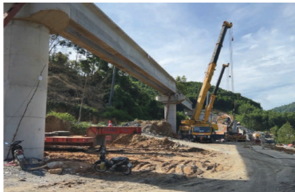
Investor: Railway Project Management Board Project name: Railway renovation in Khe Net Pass area on the Hanoi - Ho Chi Minh City railway line Contract price: 130,391 million VND Implementation year: 2024-:2025 Railway bridge project, level II
