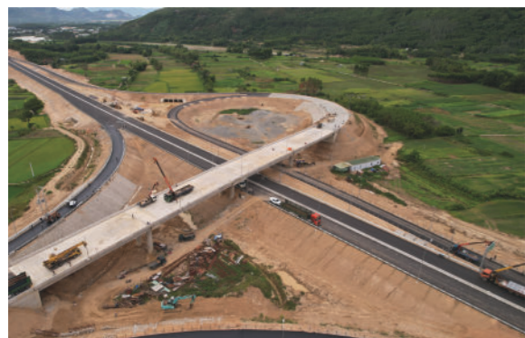
Investor: Ho Chi Minh Road Project Management Board Project name: Construction project of the North - South expressway in the East phase 2021 - 2025 Contract price: 611,761 million VND Implementation year: 2023-:2025 Road bridge project, level III
