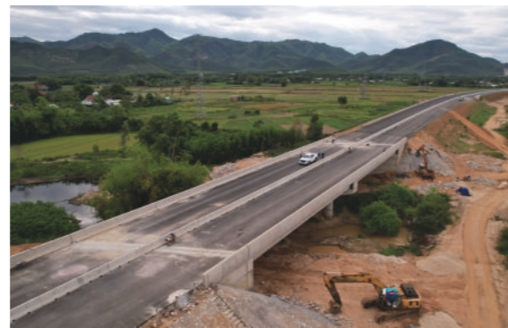
Investor: Ho Chi Minh Road Project Management Board Project name: Construction project of the North - South expressway in the East phase 2021 - 2025 Contract price: 620,994 million VND Implementation year: 2022-:2025 Road bridge project, level III
