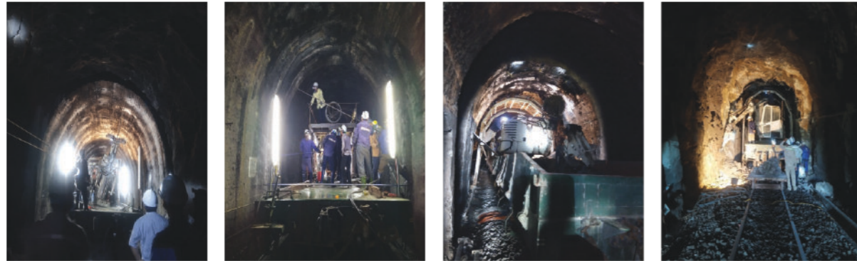
Investor: Project Management Board 85 Project name: Strengthening weak tunnels combined with opening new stations and renovating the upper-level architecture of the Vinh - Nha Trang section, Hanoi - Ho Chi Minh City railway line Contract price: 90,542 million VND Implementation year: 2020-2022 Railway tunnel project, level I
