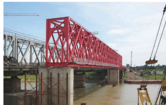
Investor: Railway Project Management Board Project name: Upgrading the Duong River waterway transport route (Duong railway bridge) Contract price: 227,814 million VND Implementation year: 2023-2025 Railway bridge project, level I
