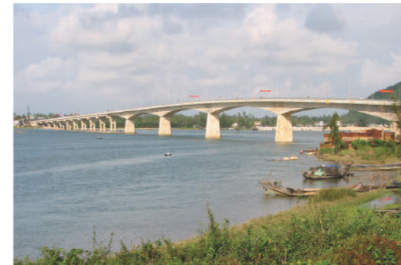
Investor: Department of Transport of Thua Thien Hue Project name: Tu Hien Bridge Km 88+600, National Highway 49B, Hue City Contract price: 40,824 million VND Implementation year: 2004-:2007 Road bridge project, level II
