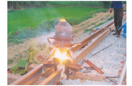
Long rail welding
